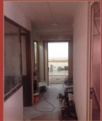
Work continues in the daughter work of Manressa
