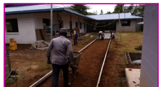
Pouring the footpaths to the classrooms
